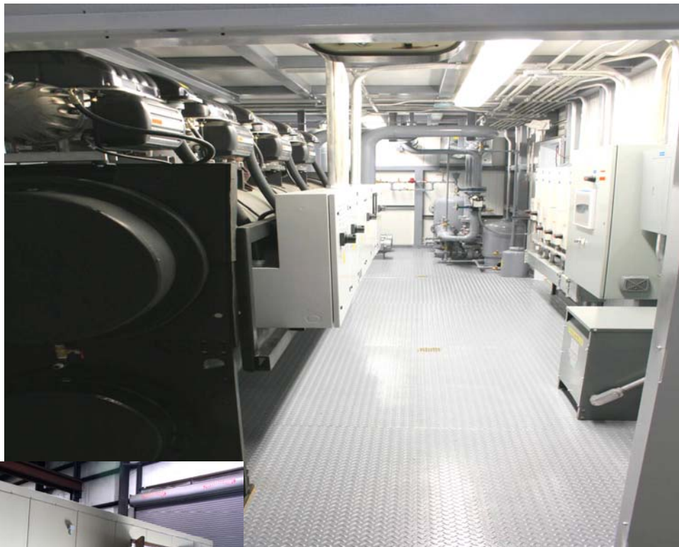
Modular Chiller Central Plant w/ Turbocor Compressor
